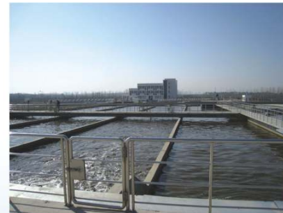
污水处理厂 Wastewater treatment plant 단지는
