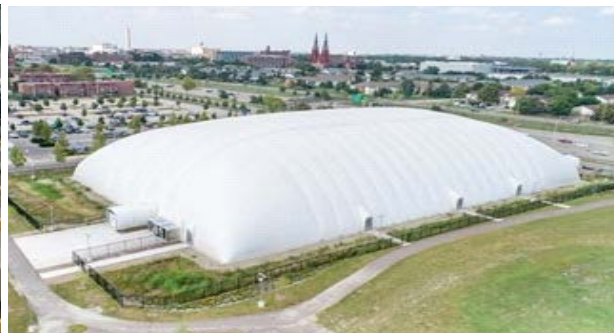
[ 집수조 덮개 설치예시#2(기타재질, air supported enclosure) ]
