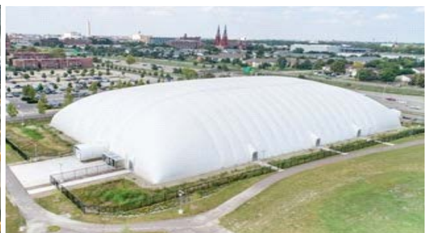
[ 집수조 덮개 설치예시#2(기타재질, air supported enclosure) ]
